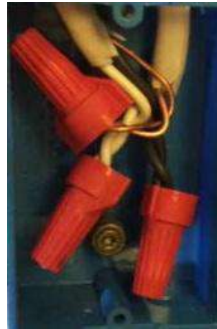
Figure 6 - Ceiling of inverter bay. Note the plastic junction box that ties the original inverted string to the PDU.
