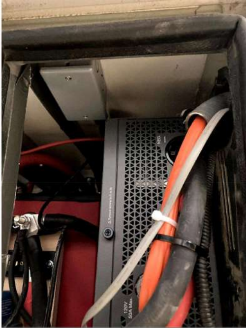
Figure 6 - Ceiling of inverter bay. Note the plastic junction box that ties the original inverted string to the PDU.
