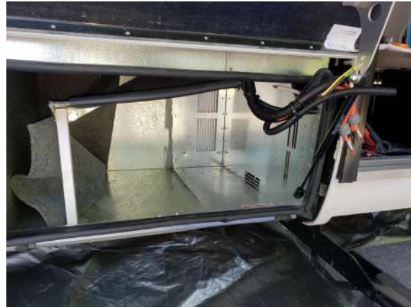
2 sides removed and propped out of the way.
