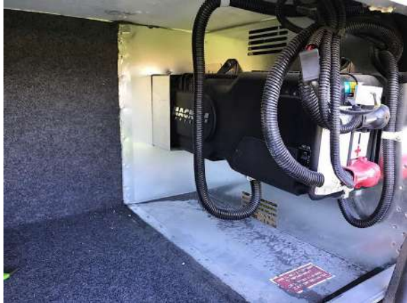
Wall completely removed.
