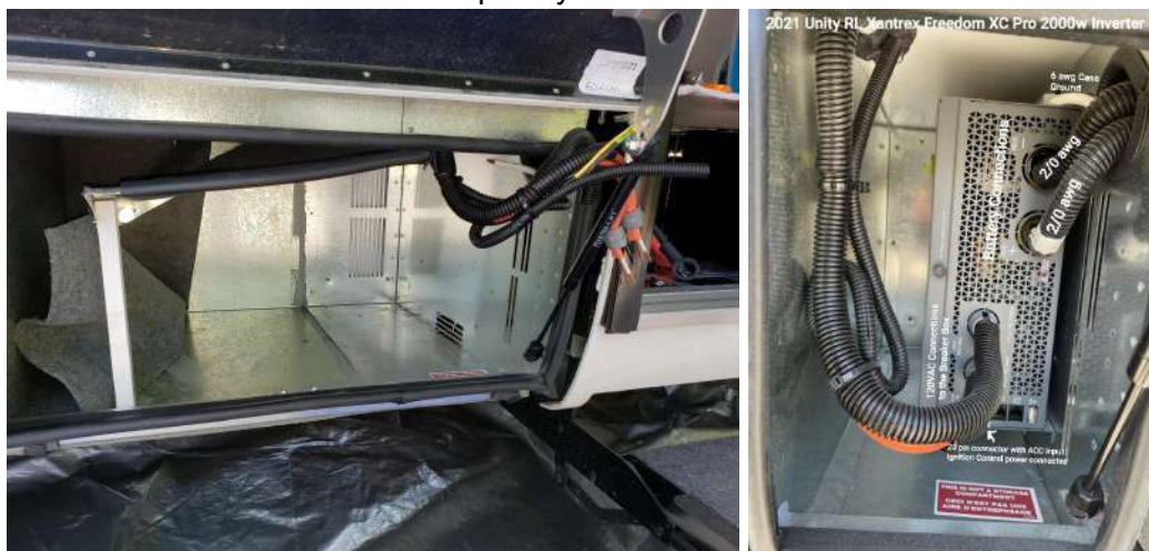
2021 Unity with inverter bay wall propped open and 2000w inverter removed
